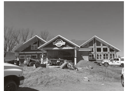
Construction approaches completion on April 22nd
