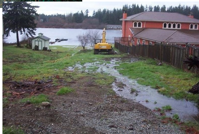
Stormwater runoff near lakeshore
